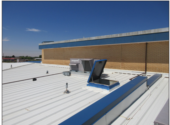
Newly Coated Roof System -
