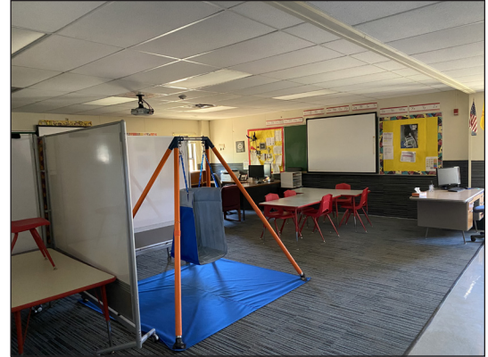
New Flooring Upgrades @ Elementary II Bldg 2015
