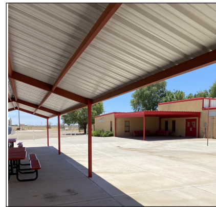
New Covered Walkway South Entry @ Main Bldg 2015
