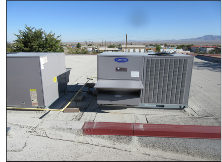
Partial Mechanical Upgrades @ DTMS
