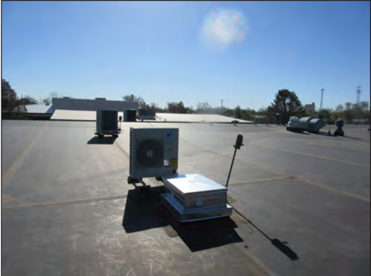
New Roofing & Mechanical Upgrades @ Elementary
