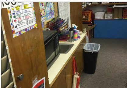
Replace casework in elementary and middle school classrooms
