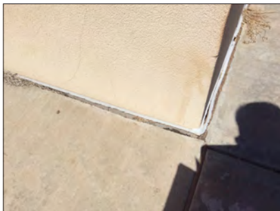
Install new expansion material and seal building perimeter
