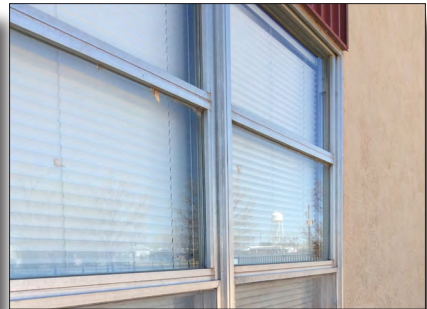
Replace windows at all classrooms
