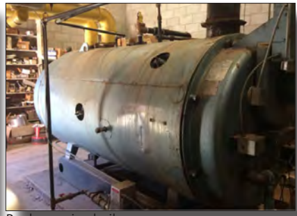
Replace aging boiler
