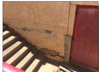
Repair stucco and replace doors to boiler room
