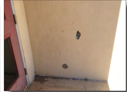
Repair damaged stucco and recolor coat
