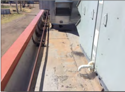
Clean debris off of roof
