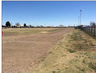
Pave track and install irrigation at baseball fields
