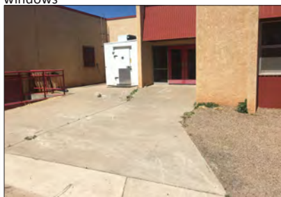
Replace spalled concrete and exterior doors & windows
