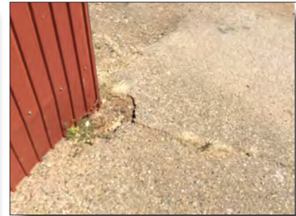
Repair building corner and asphalt - install bollards
