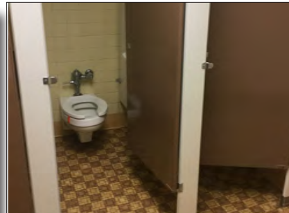
Renovate restrooms and comply with ADA
