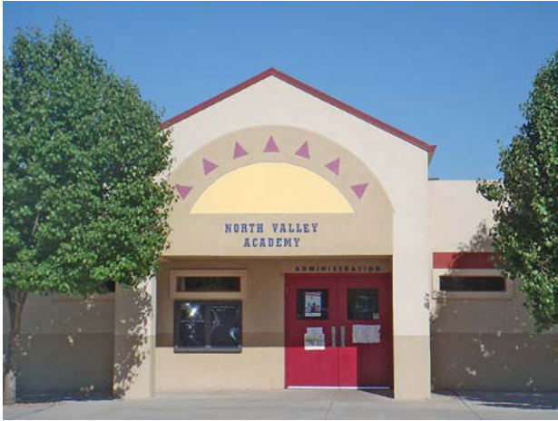
Front Entry Facade
