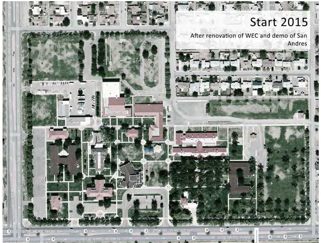
NMSBVI Campus After Renovation of WEC and Demolition of San Andres
