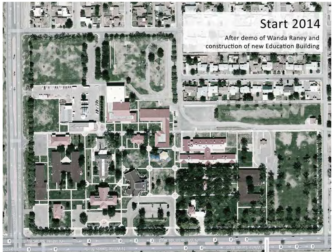
NMSBVI Campus After Demolition of Wanda Raney Building and Construction of New Education Building
