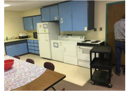
Stove is not properly vented
