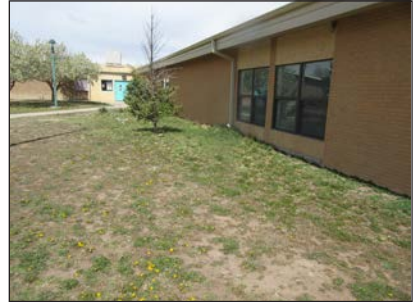
Install concrete apron around building
