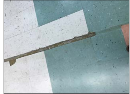
Replace VCT throughout
