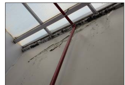
Replace skylights & repair wall damage
