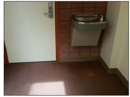
Replace water fountains
