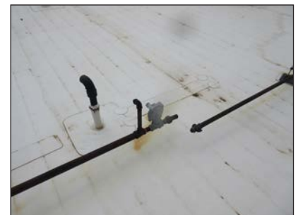
Reconnect gas lines & test for leaks-multiple locations
