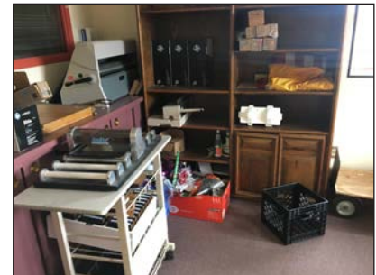
Replace casework throughout
