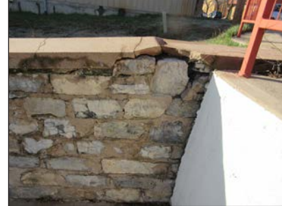
Repair rocks at retaining wall at south side of Gym
