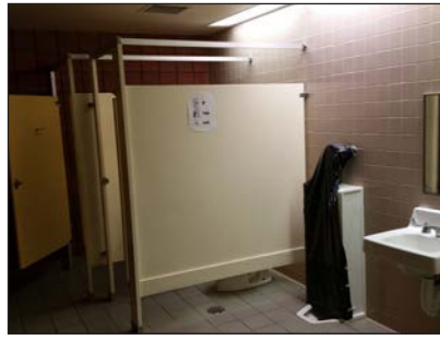
Renovate all restrooms
