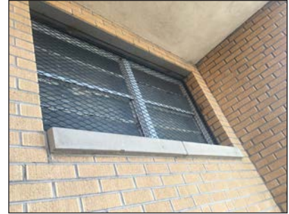
Replace all exterior windows-single pane
