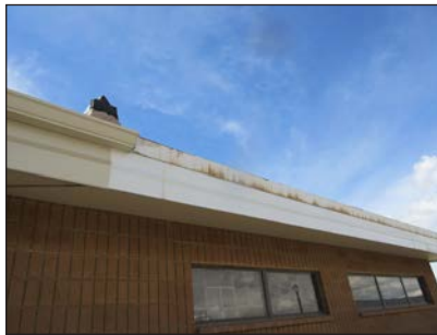
Replace missing gutters
