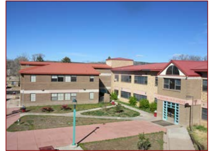
Main Academic Building & Student Commons
