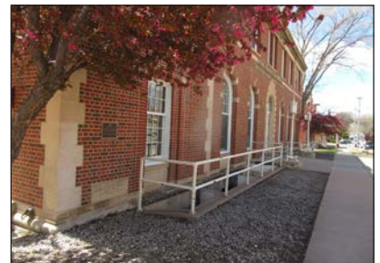
Main Entry to Building
