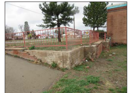
Replace retaining wall
