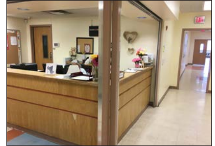
Provide secure admin & main entry
