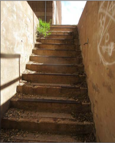
Replacement access stairs to basement & provide handrails
