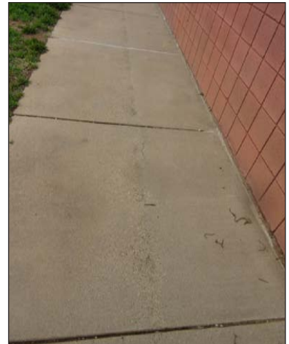
Reseal building perimeter at sidewalks
