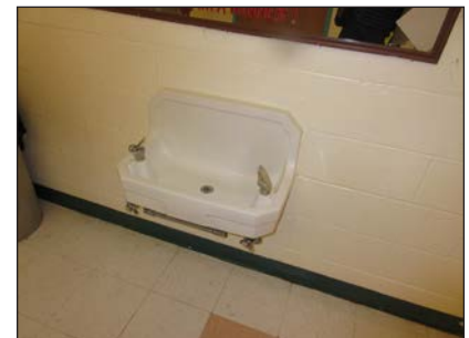
Replace water fountains
