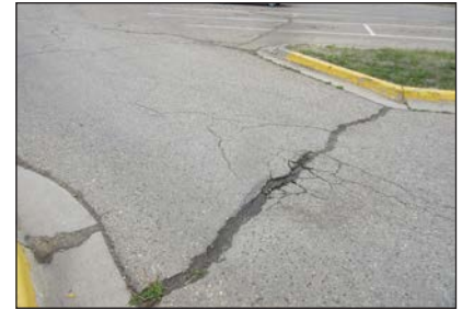
Repair all cracks & resurface parking lot
