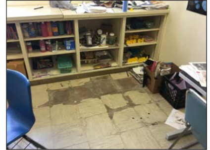
Replace flooring & casework in all restrooms
