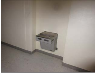
Replace water fountains
