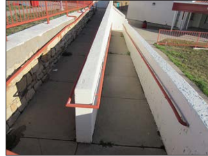
Stabilize retaining wall & repair ramp
