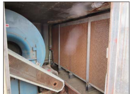
Replace cooling system
