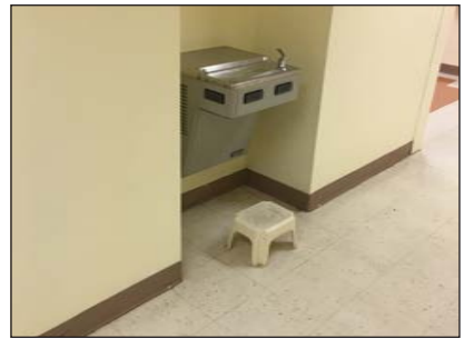
Replace water fountains & comply w/ ADA
