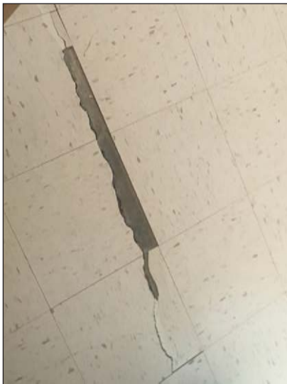
Replace VCT flooring
