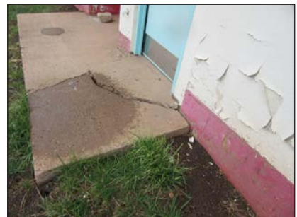
Replace broken concrete stoop
