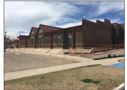
Media Center / Science Building
