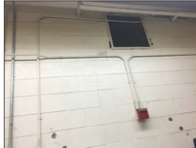
Replace ventilation system & repair walls
