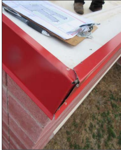
Install caulking at turn seams
