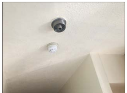
Replace light fixtures
