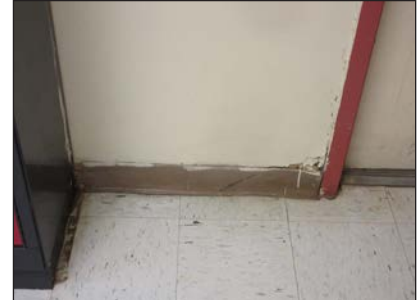
Replace flooring & wall base
