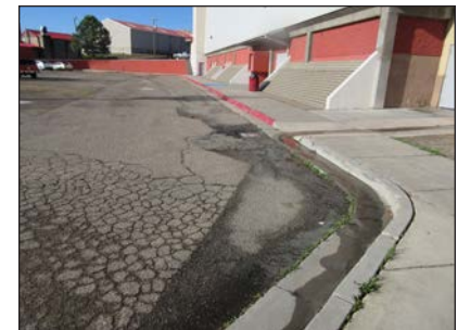
Repair [saving & resurface
