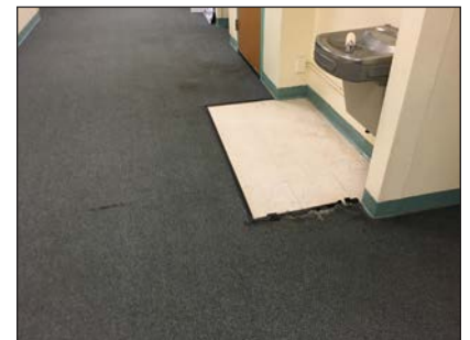
Replace carpeting throughout
