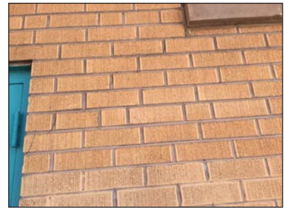
Repair & tuck-point exterior masonry
