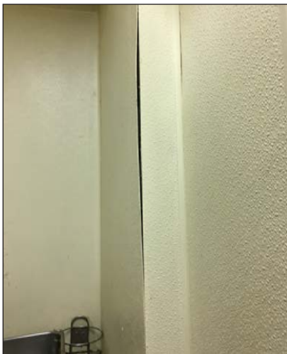
Install corner guards throughout
