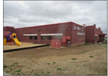
Drainage improvements needed around perimeter
