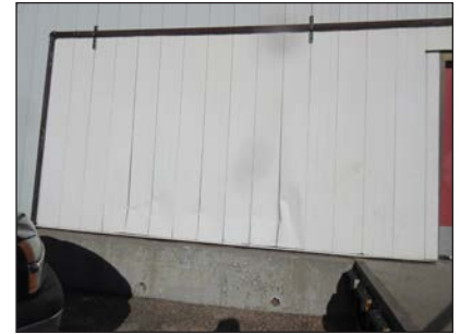
Replace damaged wall panels
