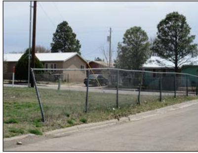
Replace all damaged site fencing
