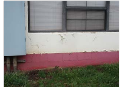
Install concrete apron around perimeter of building
