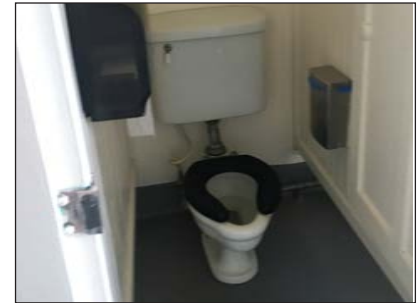
Original Plumbing Fixtures
