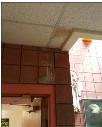
Repair interior walls/ceilings
