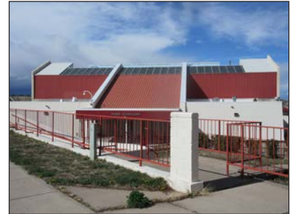
Marr Gym - Repaint metal handrails
