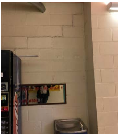
Structural repairs in corridors
