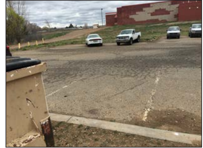
Repair & resurface parking lot
