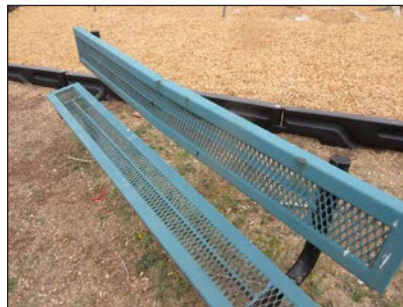
Replace damaged benches
