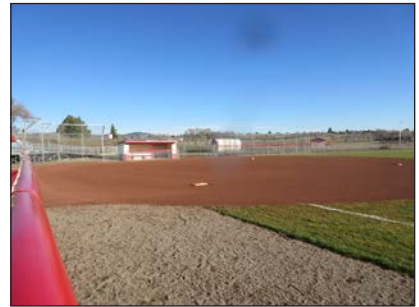
Field upgrades completed
