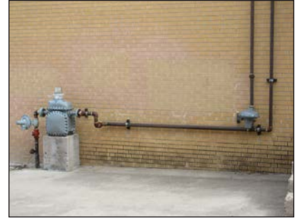
Clean masonry & tuck-point exterior walls
