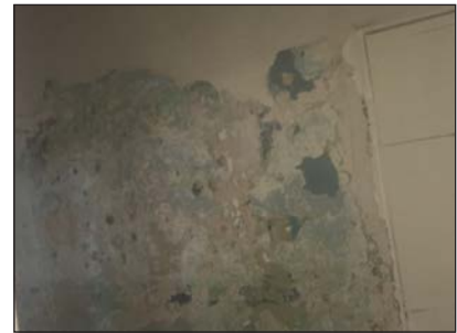
Repair wall damage at fire riser room
