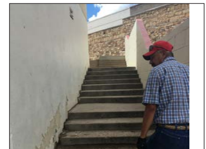
Repair/repaint walls & install handrails
