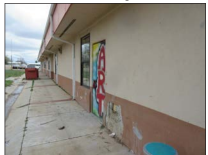
Repair stucco & recolor coat
