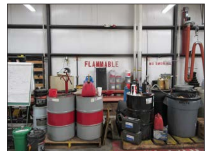
Due to amount of flammable material, a separate room enclosure may be required code analysis
