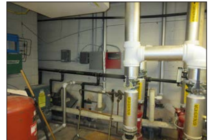
New boiler system
