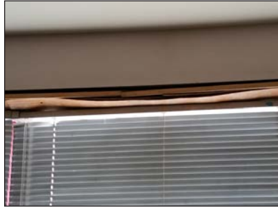
Repair window header
