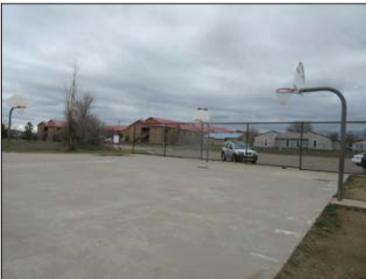
Repair basketball courts
