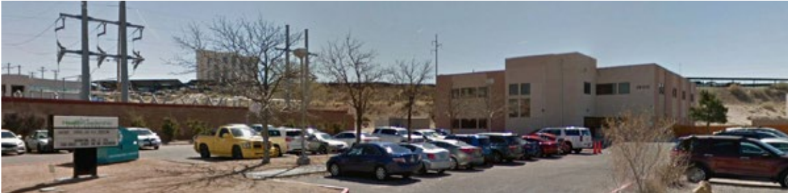
HLHS Current Leased Facility
