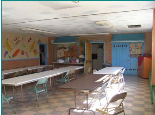
Existing multipurpose room.
