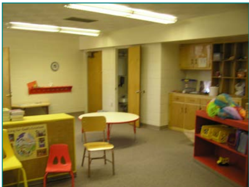
A typical classroom before restoration.
