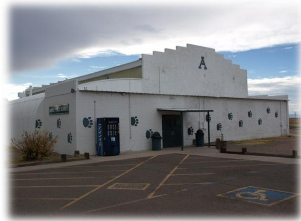
APS MIDDLE SCHOOL GYMNASIUM
