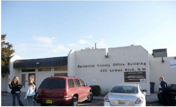
Front (north) side of building
