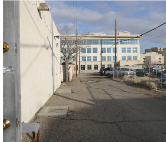
Back (south) side of building at alley
