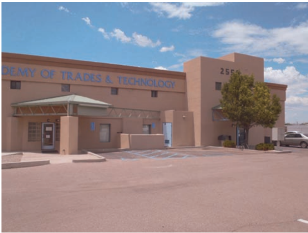
Front Entry Facade
