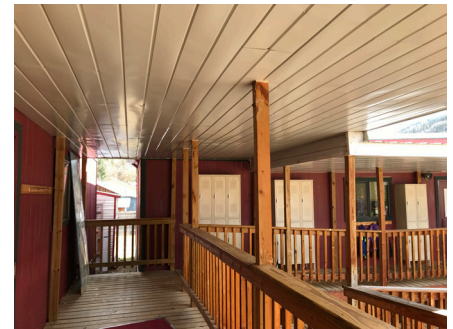
Covered exterior walkway at portable
