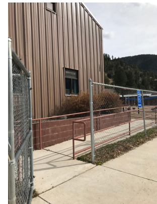
Improve signage and fencing
