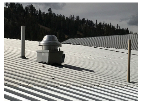
Roof detail at potential leak source
