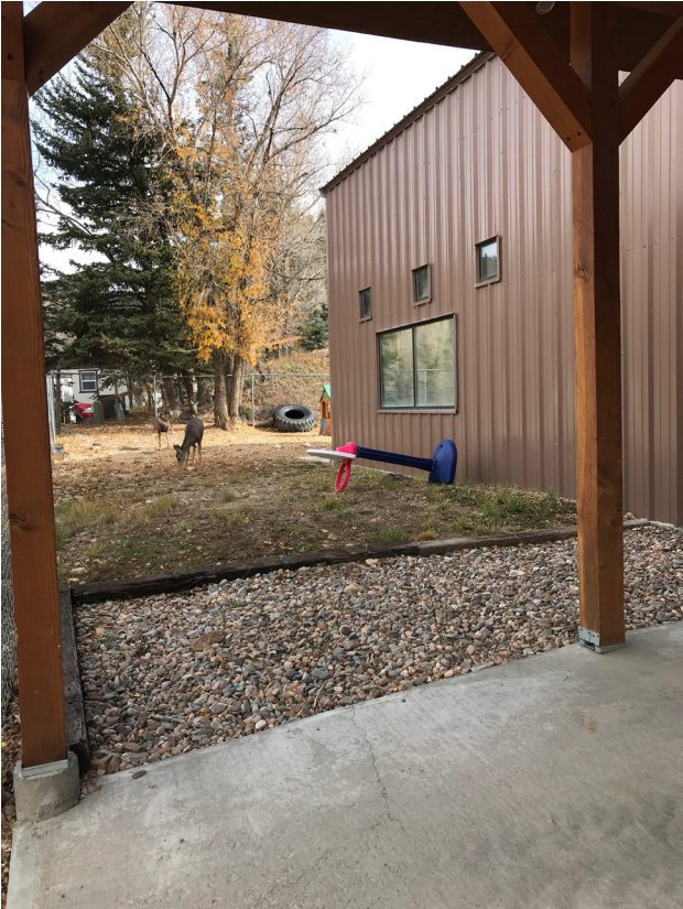
View at Entry to pre-K playground
